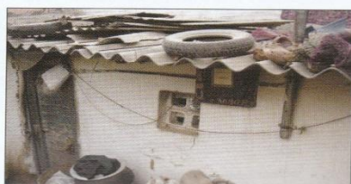
Typical exterior condition of AC roofing in New Lingarajapuram. Note the broken AC roofing sheets, low roof height and the ventilation 'window' – a typical size in the homes of New Lingarajapuram.
