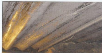
Charred and cracked AC roofing after long-term use (same dwelling as above).
