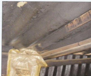
Pitting and smoke damage on AC roofing after long-term use (same dwelling as above).
