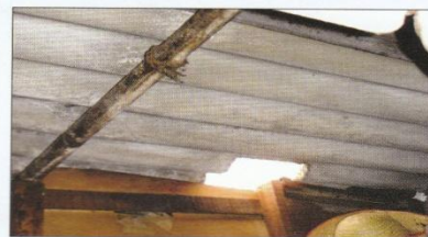
Homemade skylight cut into AC roofing, the cutting of which releases harmful chrysotile fibres into the environment. The roof has been previously painted with white emulsion paint which deteriorates rapidly, often showing signs of discolouration and mould. Note the contrast in ceiling colour when compared to white ceiling fan (top right).
