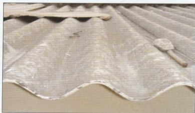
Exterior AC roofing in reasonable condition. Note surface weathering.
