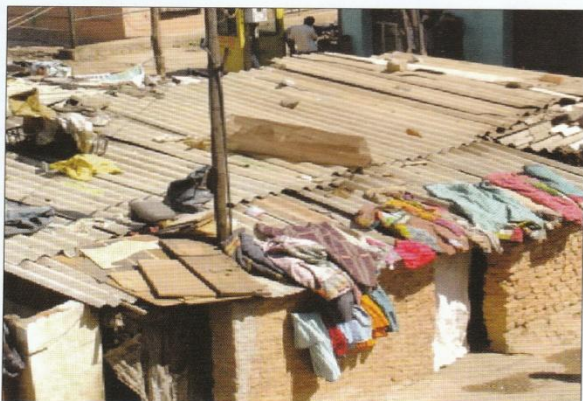
Typical AC roofing in New Lingarajapuram, Bangalore. Note lack of ventilation apart from that available by using the doorway.
