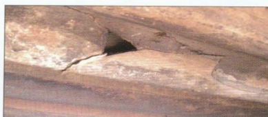
Smoke damaged and cracked AC roofing (same dwelling as above).
