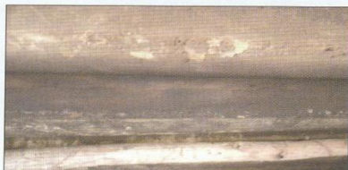
Flaking and pitted AC roofing, resulting from smoke damage. House was newly built and had been occupied for one year at the time of survey.
